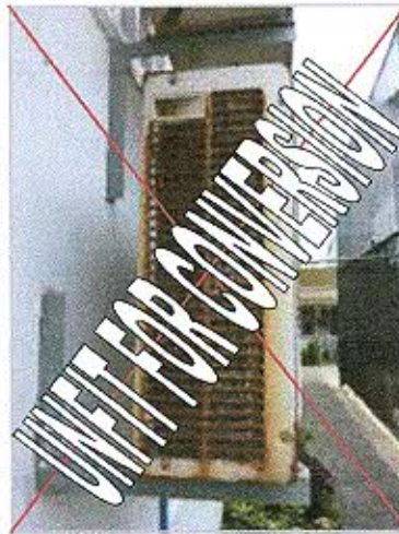
Figure 3-6: Example of AC system that is unsuitable for conversion
