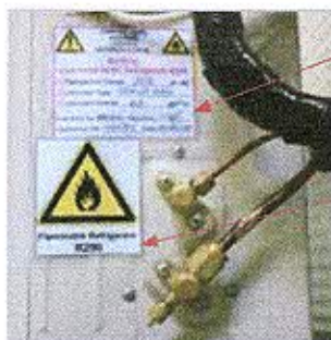
Figure 3-25: Labeling of the outdoor unit
