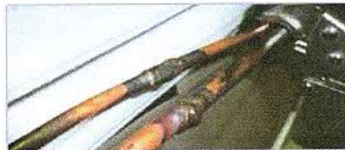
Figure 3-12 Removal of mechanical connections by joining tubes with brazing
